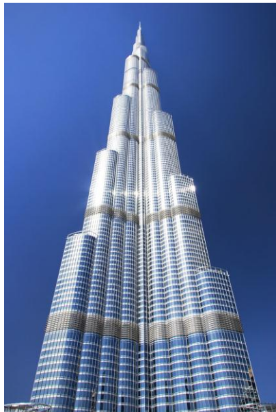
Guardian's SunGuard glass on the world's tallest building, the Burj Khalifa in Dubai, U.A.E
